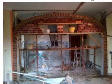
Liebenow kitchen during renovation
