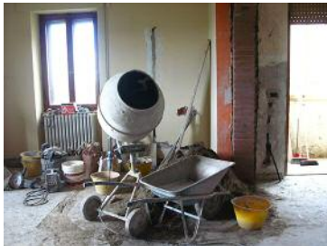
Liebenow living room during renovation
